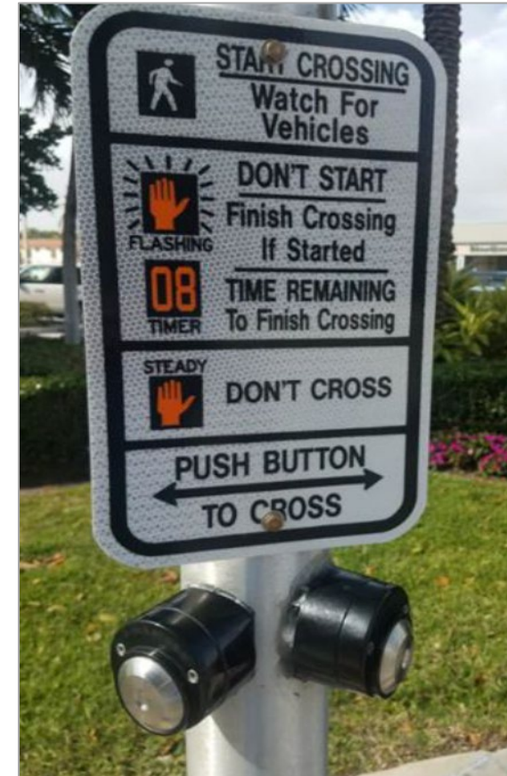
Installing pedestrian countdown signal features
